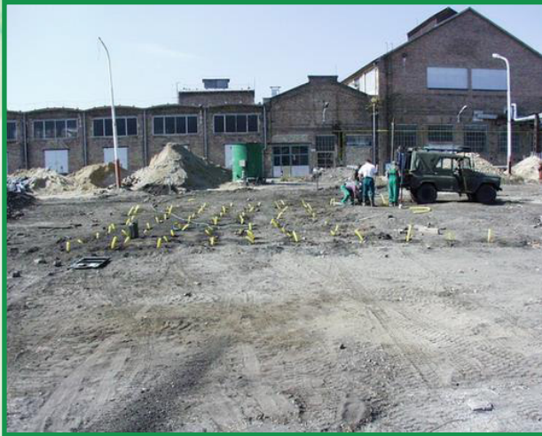
fill-up of the holes with enzyme
