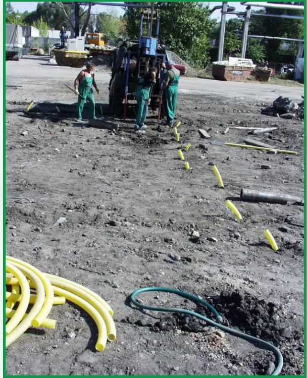
installation of perforated pleated hoses
